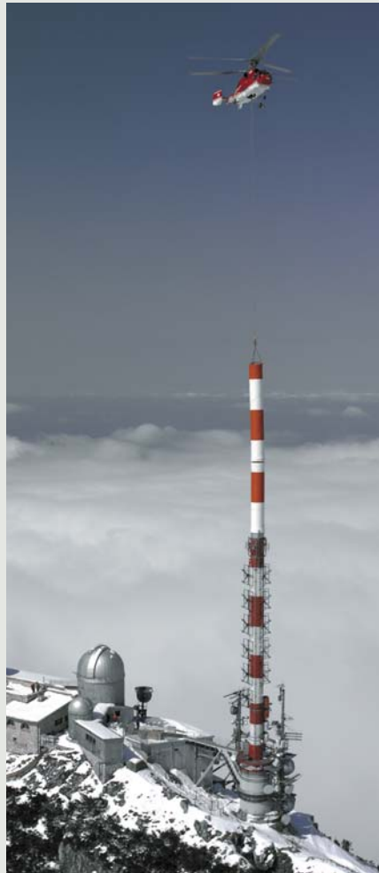
Wendelstein, Bavarian Alps Erecting new radome with DVB-T antennas from KATHREIN
