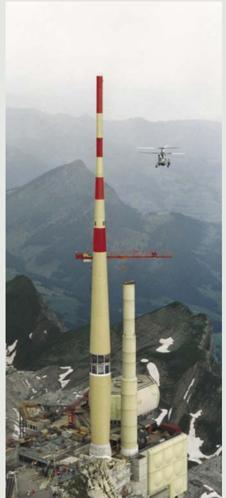
Säntis, Switzerland · 126 ft. self-supporting GRP cylinder on top and GRP panels with a height of 219.5 ft. beneath
