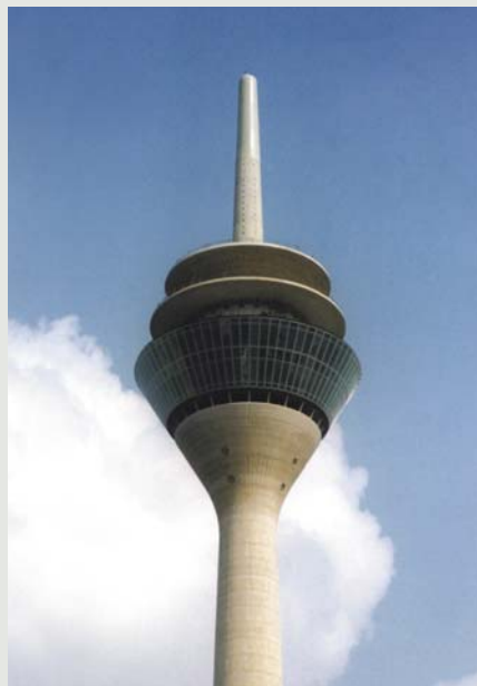
Düsseldorf, Germany · Conical GRP cylinder (1981 – 2004) Diameter 9.9 – 13.1 ft. · Length 52.5 ft.
