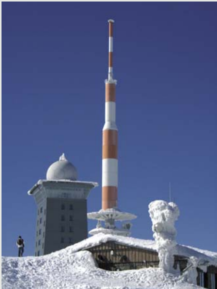
Brocken, Germany · Cylinder, dia. 5.25 ft., height 75.5 ft. · Panels, dia. 14.1 ft. and 21.3 ft., height 55.8 ft. and 118.1 ft.
